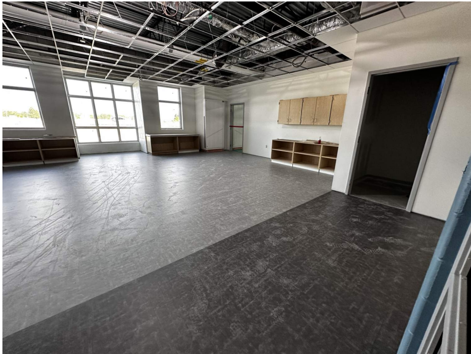
LVT flooring installed in classroom.
