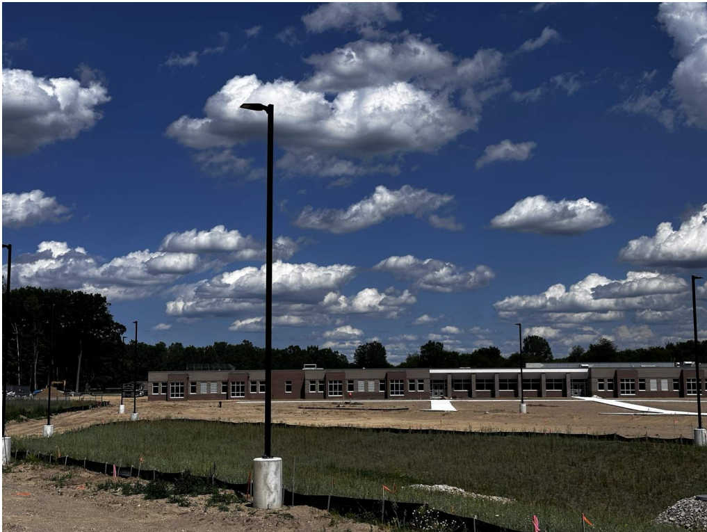
Light poles installed along bus lot drive on west side.
