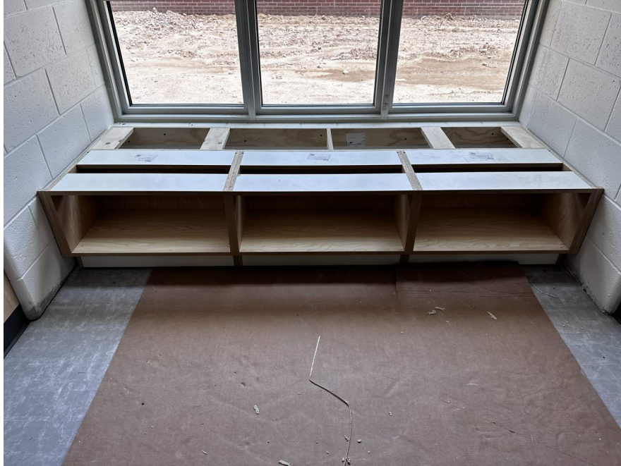
Bench install at window of classroom.
