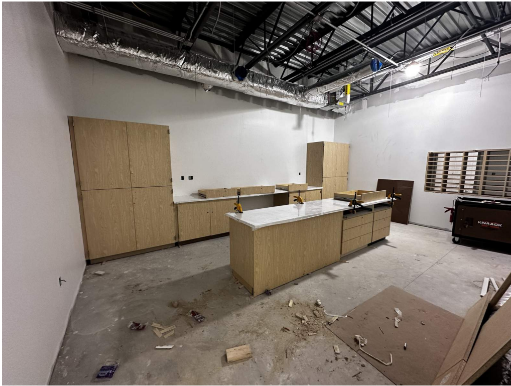
Casework in office workroom.
