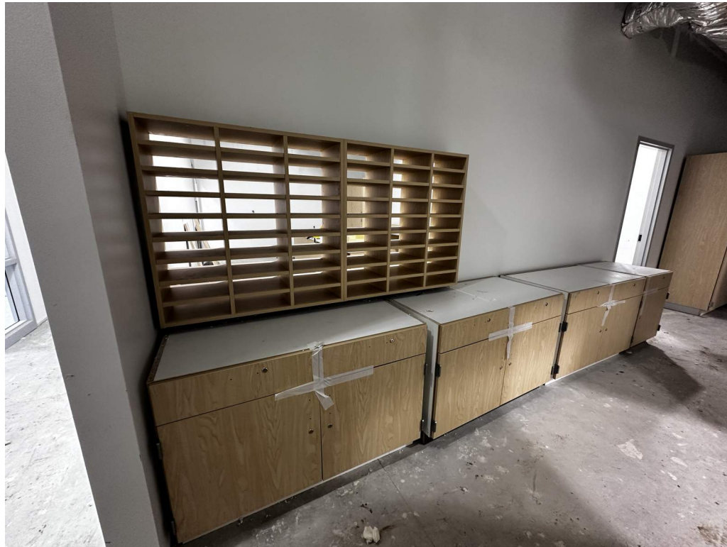
Casework and passthrough cubbies in main office.
