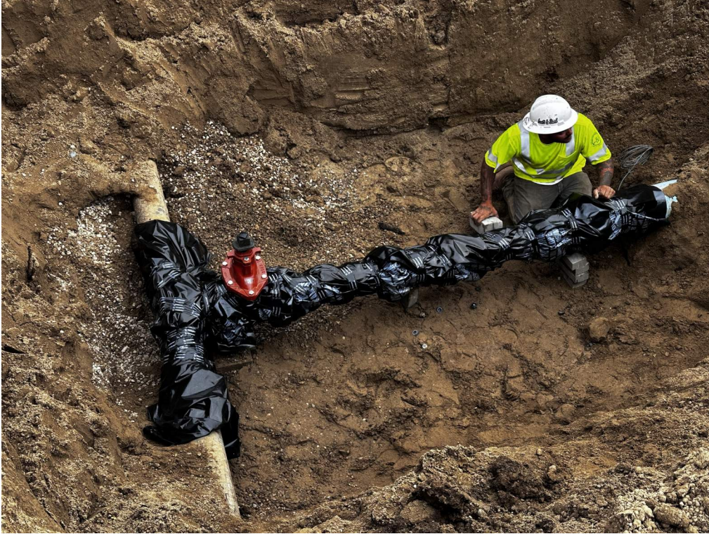
North water connection being made.
