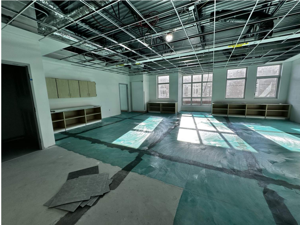
Floor prep before flooring install.
