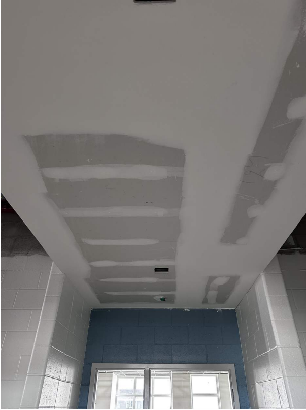
Soffit finishing outside of classroom.
