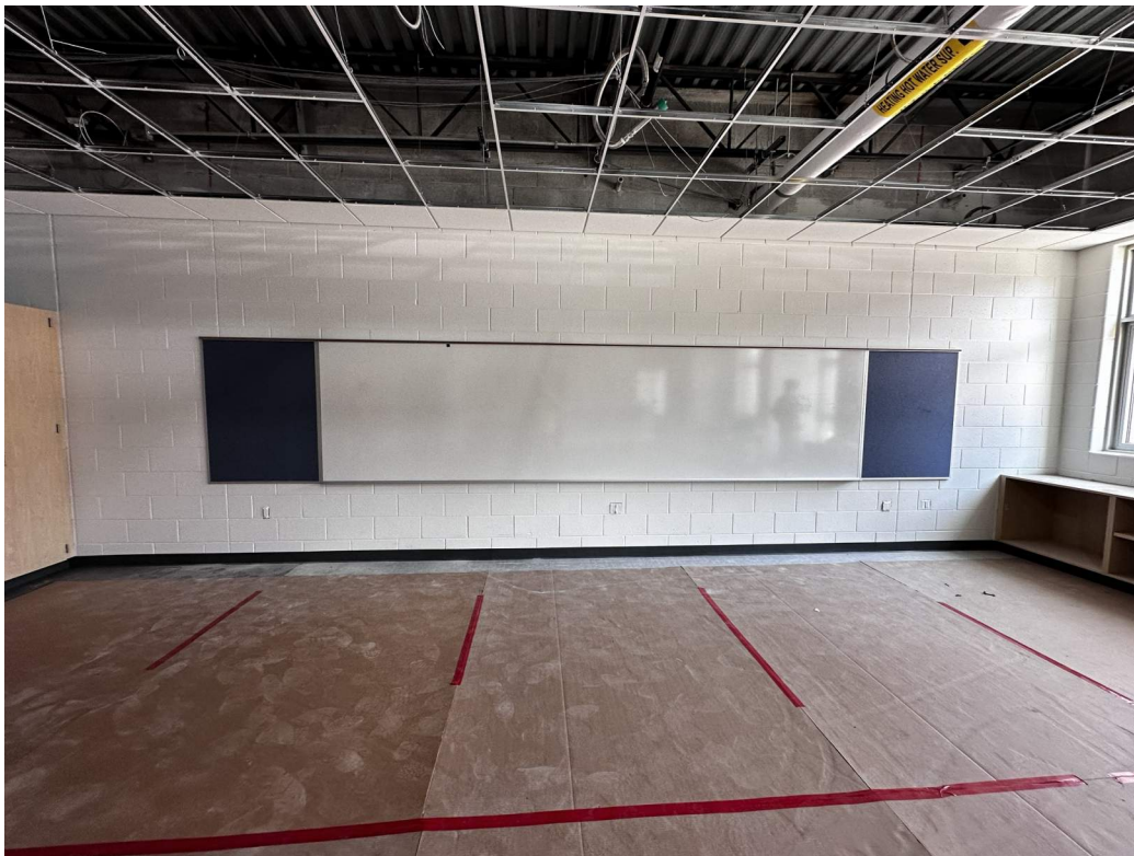
Tack board and marker board install in classroom.
