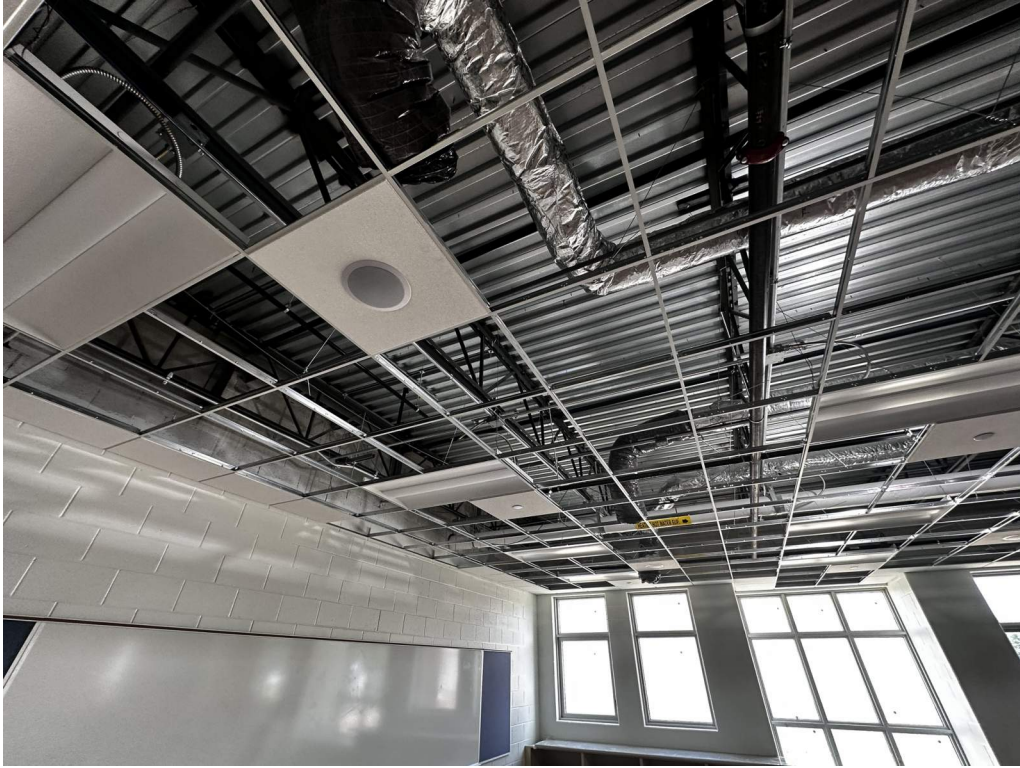
Light and speaker install in classroom.
