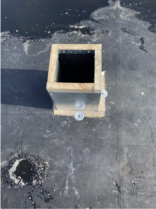
Pitch box install in progress on the roof.
