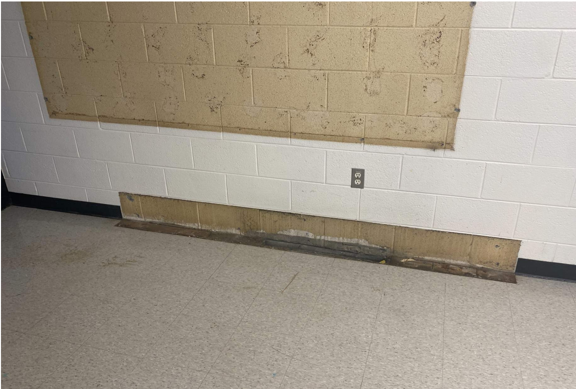
Tackboard and floor register demolition.
