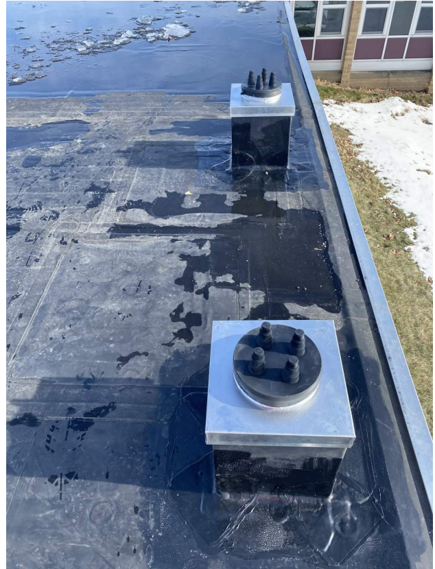
Install of pitch boxes complete on the roof.
