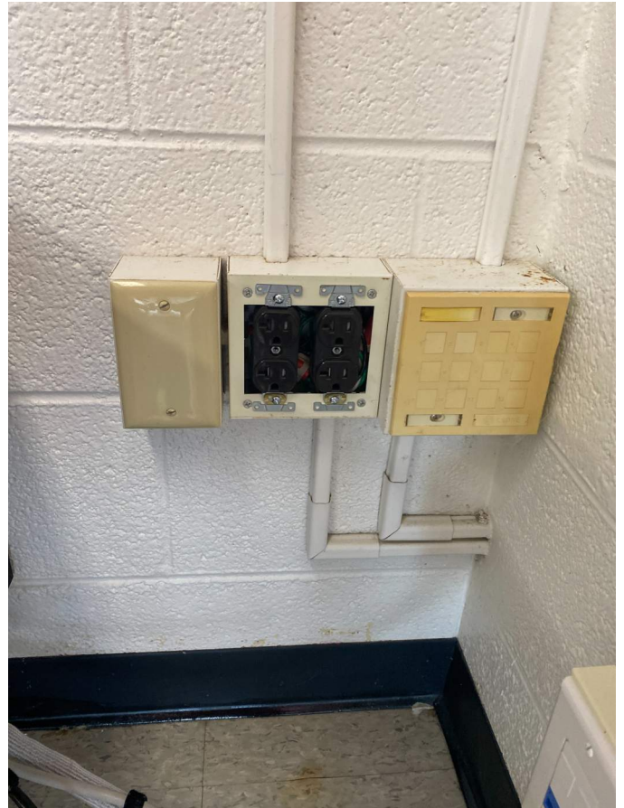
Double duplex receptacle replacement.
