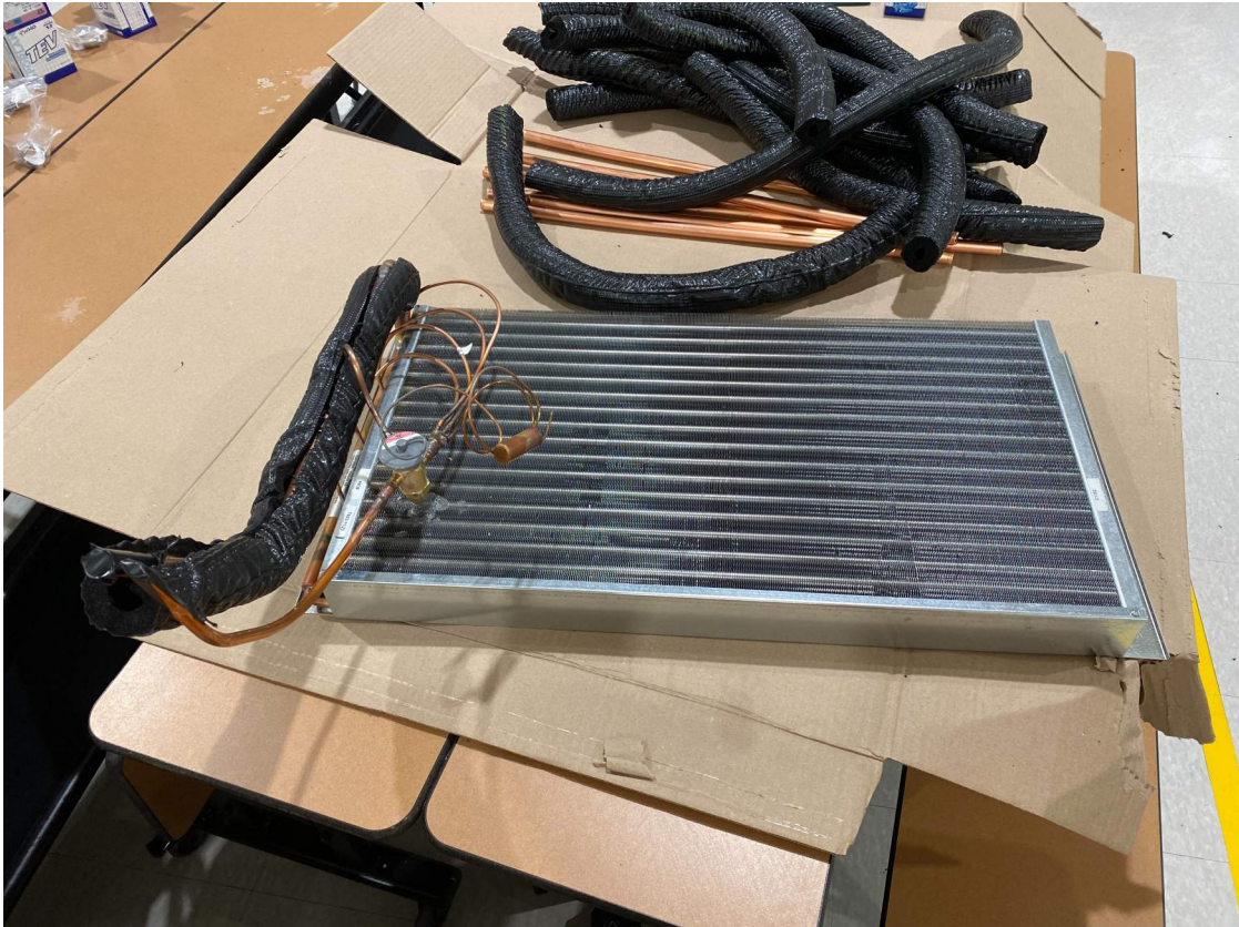
Coil removed from unit ventilator.
