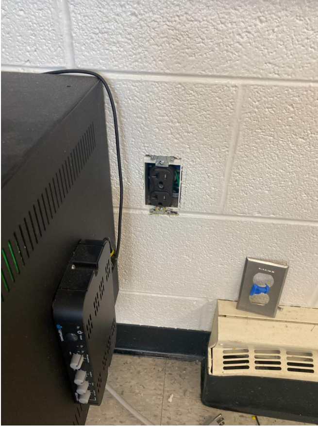
Single duplex receptacle replacement.
