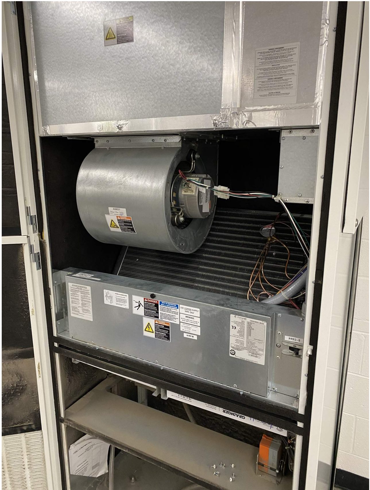
Open unit ventilator preparing for coil replacement.
