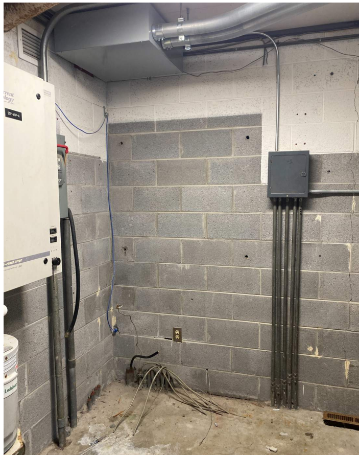
Demolition of existing electrical components.
