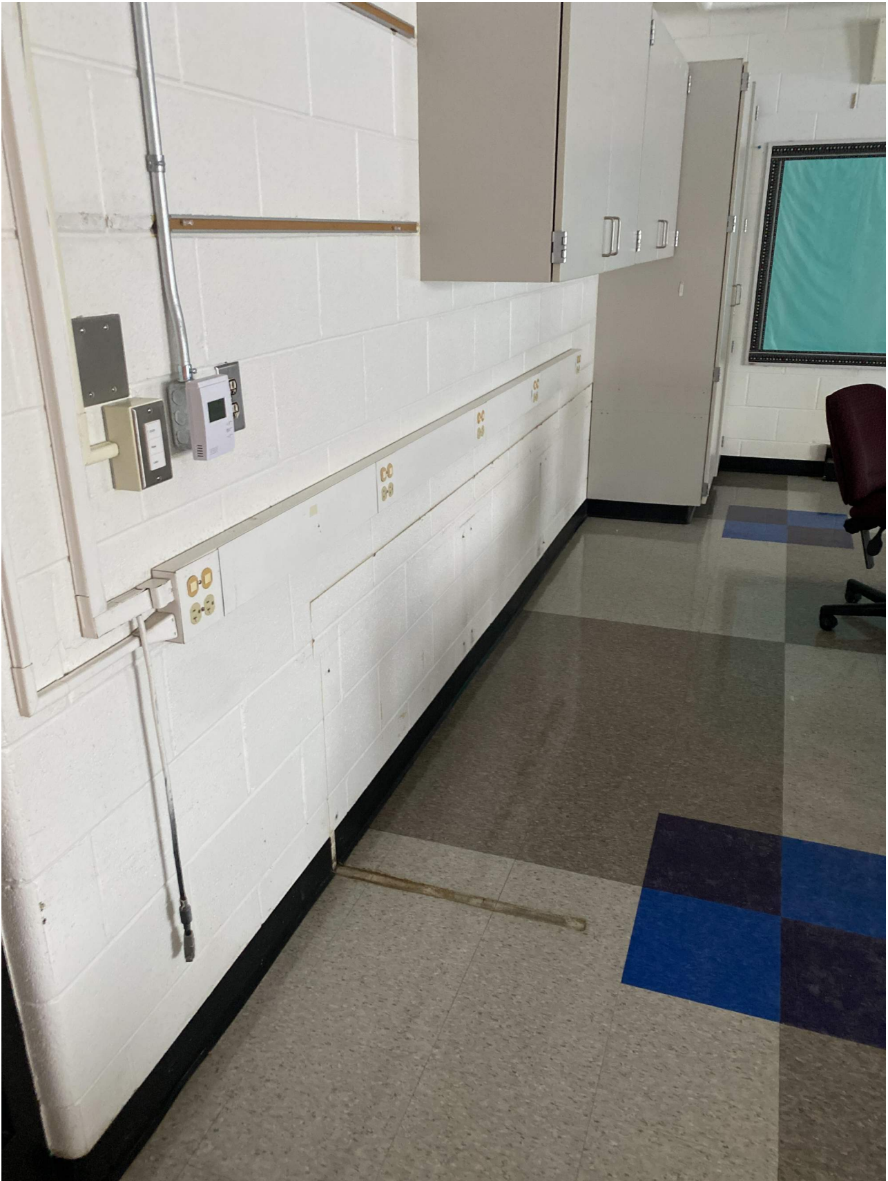
Counter top and anchor removal from classroom.
