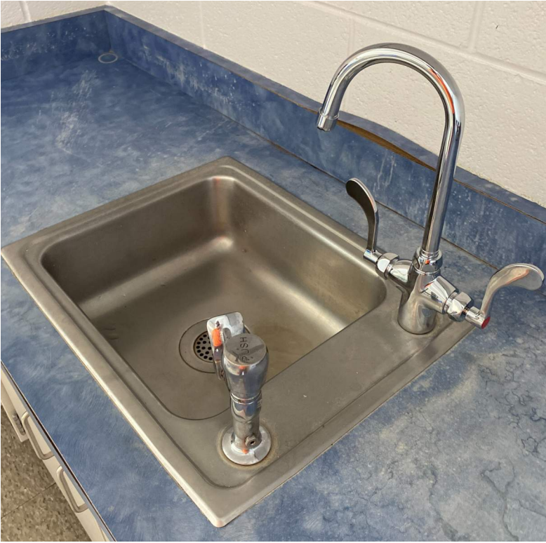
New sink faucet installed.
