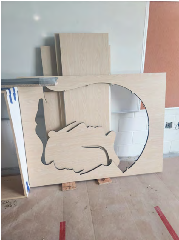
Gladiator head millwork panel prior to install.
