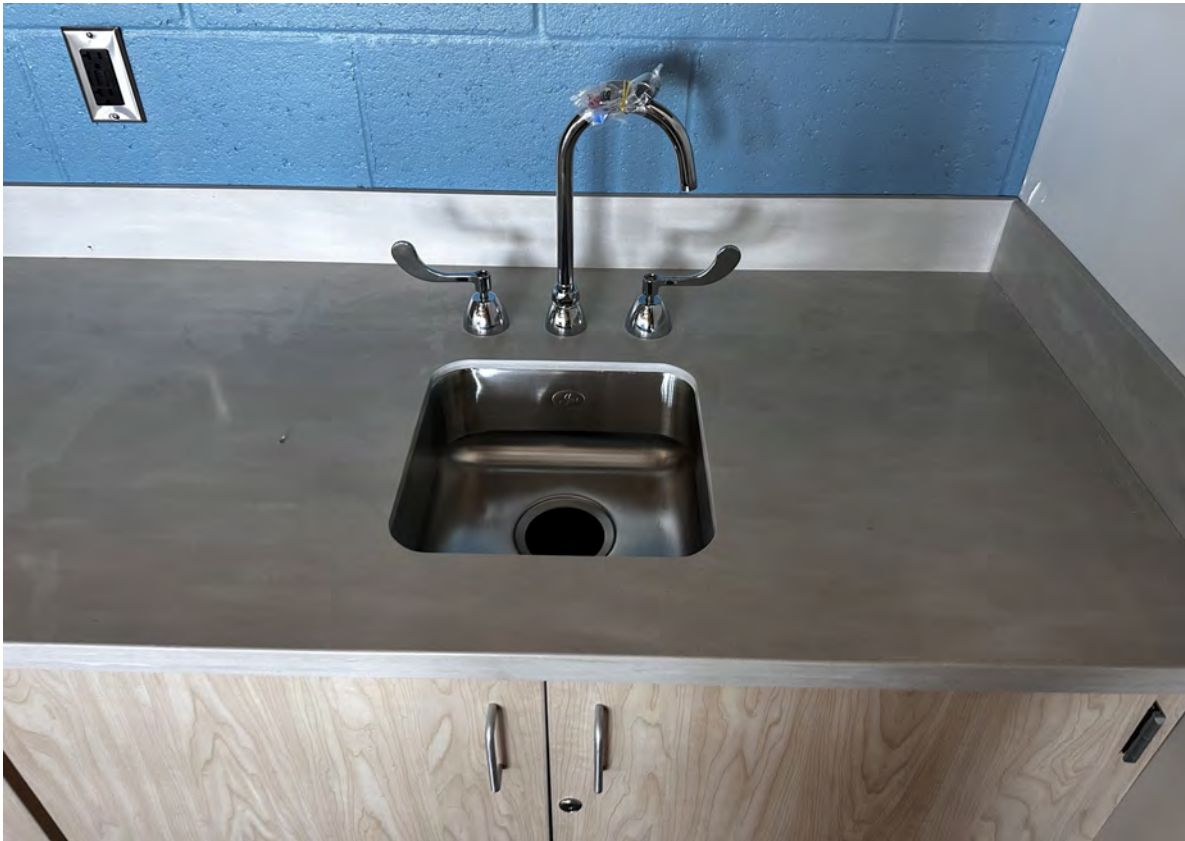
Sink installed in music room.
