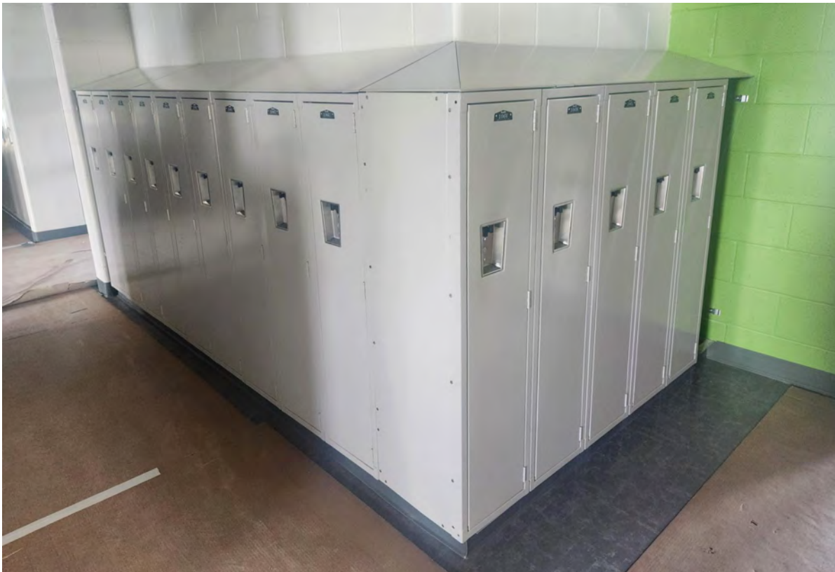
Hall lockers installed with sloped tops and numbers.
