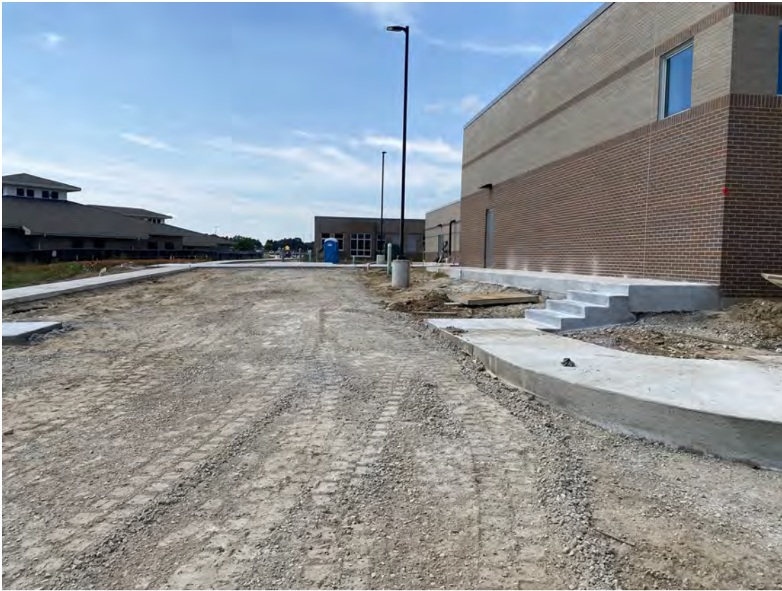
Concrete walks and stairs on the south side of the building.
