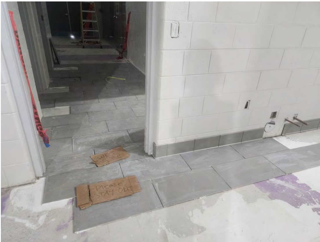
Floor tile install in the kitchen.
