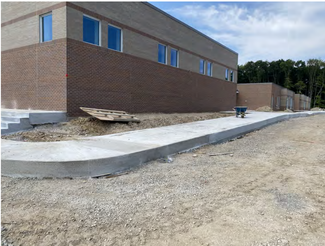
Concrete walks on the south east corner of the building.
