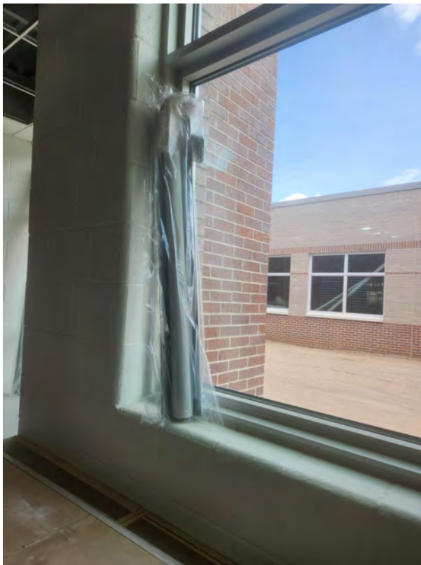
Window shade staged for install.
