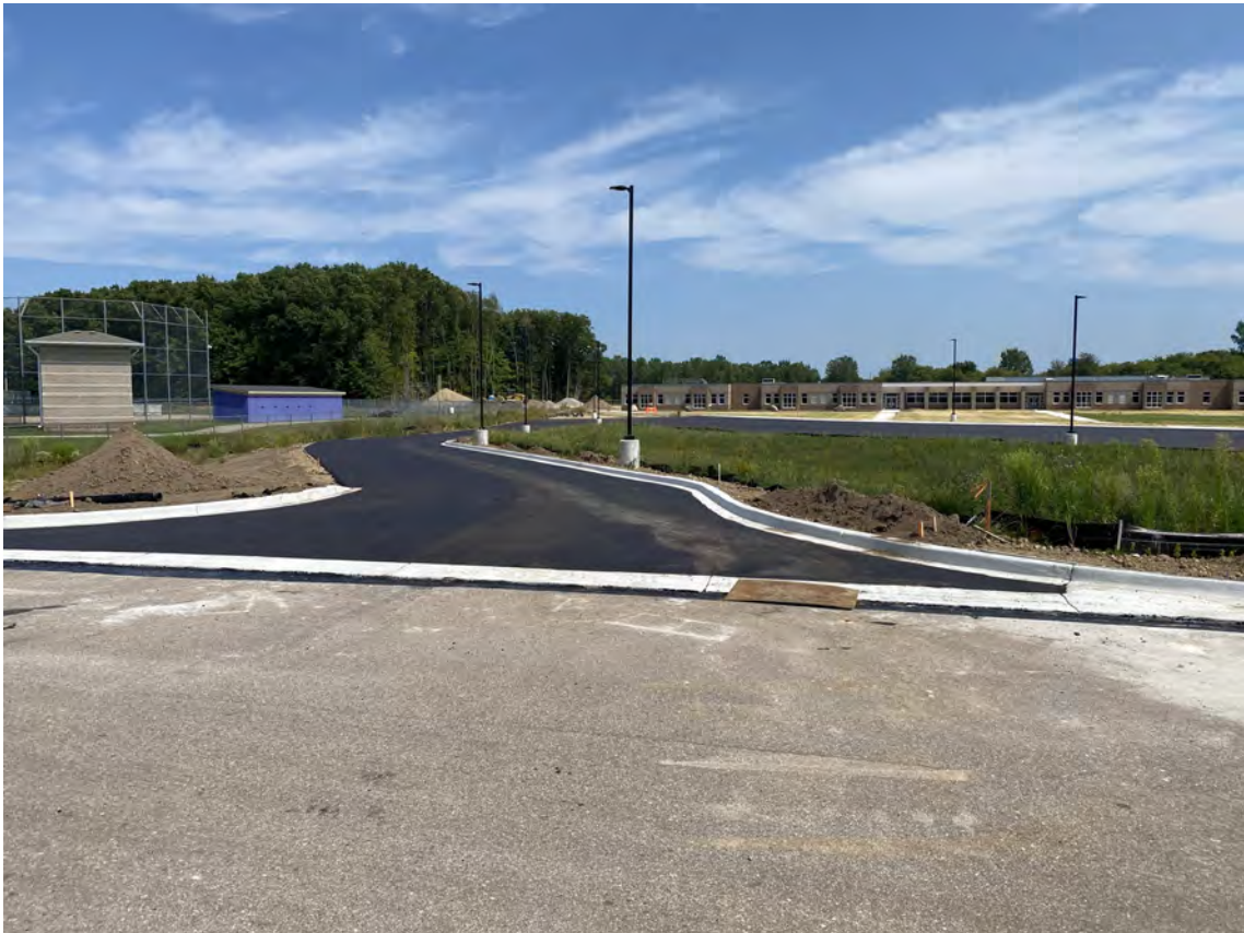
Bus lot asphalt prior to striping.
