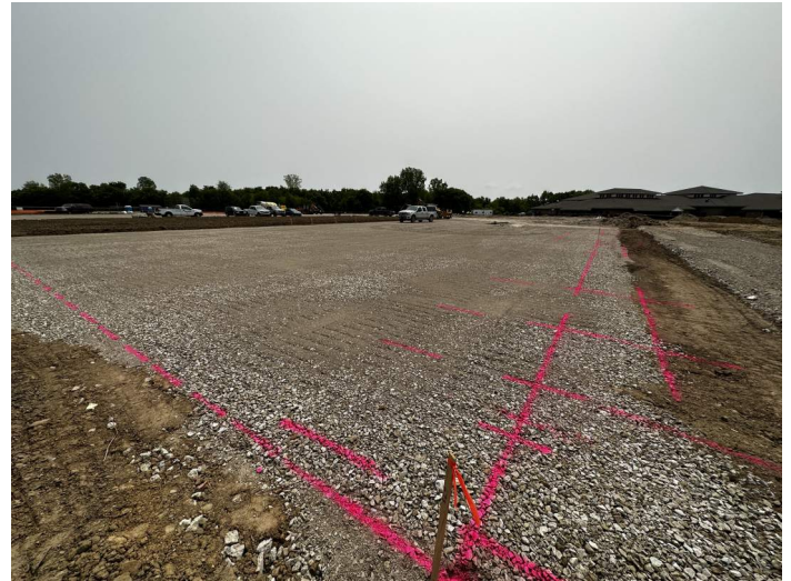
Building Pad marked with layout paint in preparation for foundations (complete).
