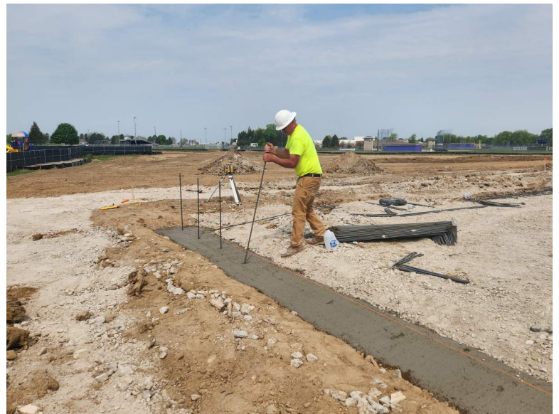
Vertical rebar install into foundations (complete).
