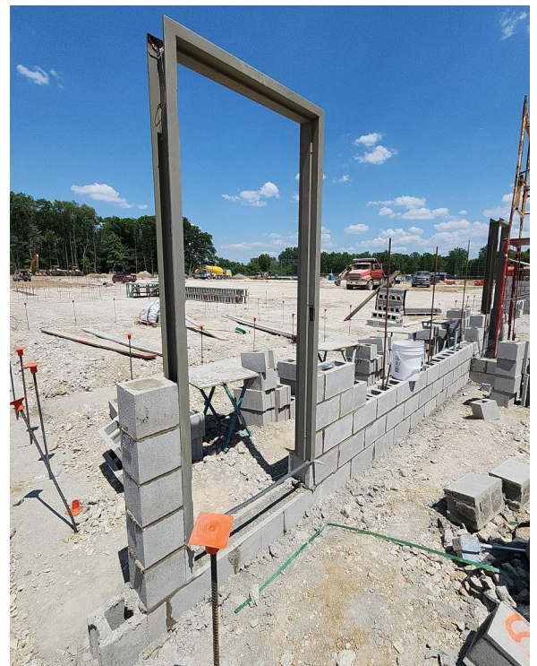
Hollow metal frame installation (in progress).
