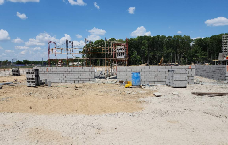
Masonry on west side of building (in progress).
