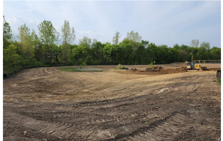
Grading at East detention basin (complete).
