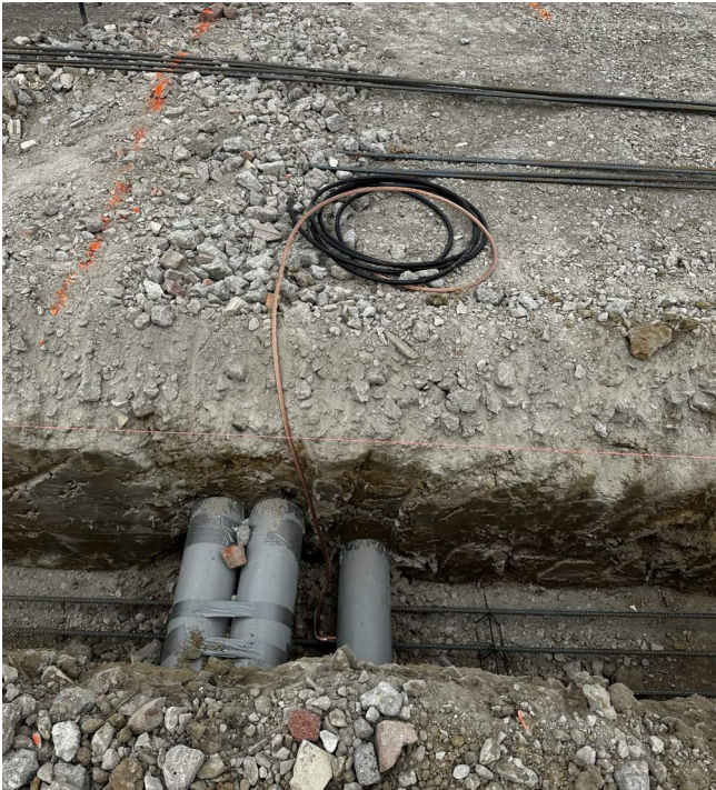
Electrical conduit install prior to foundation pours (complete).
