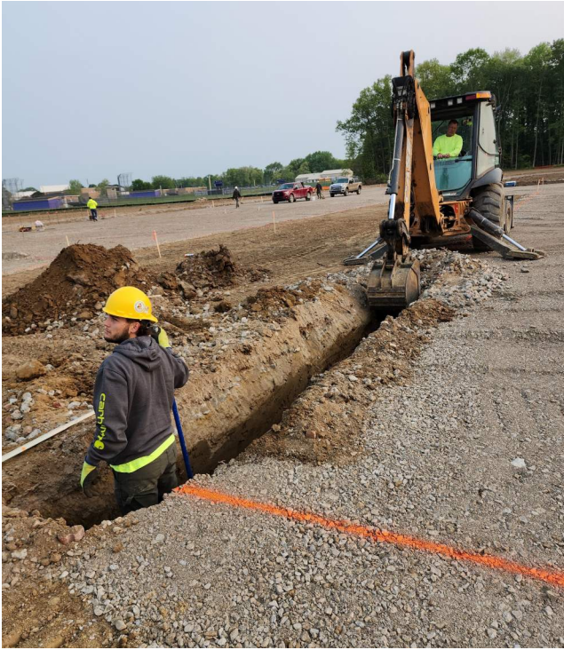
Trench digging for foundations (complete).
