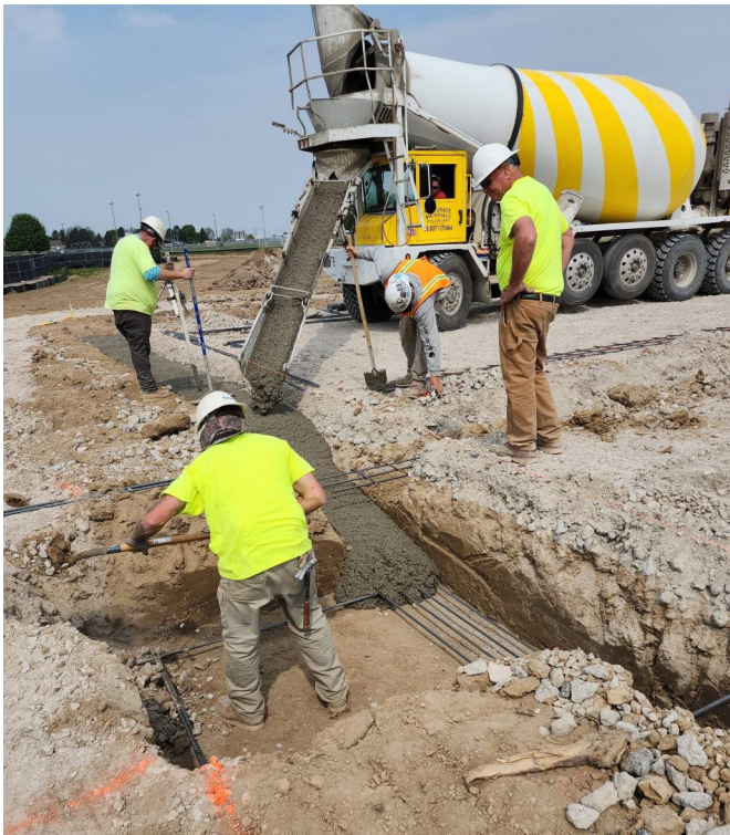
First concrete pour for foundations (complete).
