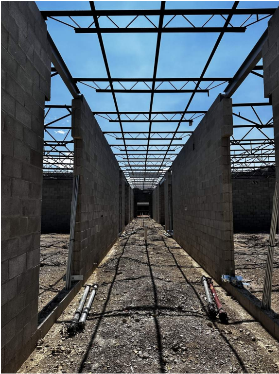
Joists set in a hallway.
