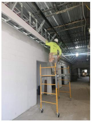
Drywall install at corridor soffit.
