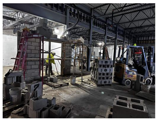
On slab masonry wall in progress in cafeteria.
