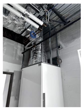
Ducting to vertical unit ventilator in classroom.
