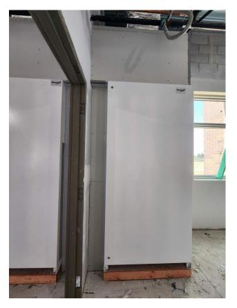
Drywall bulkhead and wing wall near vertical unit ventilator.
