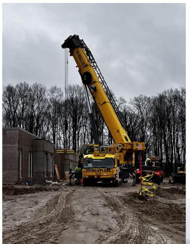
Crane used for RTU lift onto roof.
