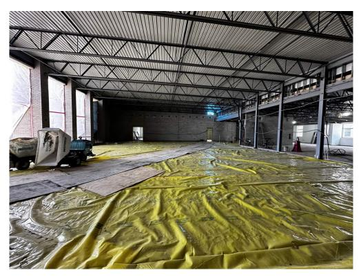
Vapor barrier installed in cafeteria prior to concrete pour.
