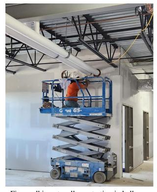
Fire caulking at wall penetration in hallway.
